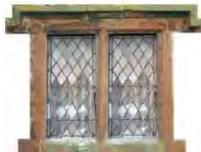
16 & early 17 century • stone mullioned • diamond leaded fixed lights
