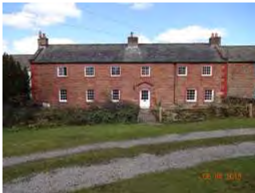
Figure 5 The grade II listed Midtown Farmhouse is an example of a building fronting the village green with a small front garden and stone boundary wall
