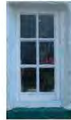
Many 16 and 17 century formerly leaded or unglazed windows have now been replaced with timber windows
