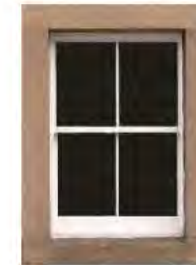
Mid to late 19 century Victorian sash 4-paned with horns
